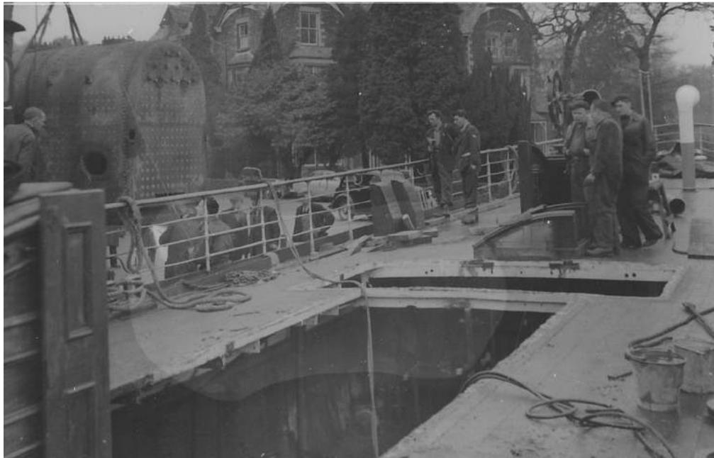
*The Windermere ships carried large single side-fired loco-type boilers. That from 'Tern' is lifted out and lowered on to a lorry on the wharfside. The unusual horizontal non-condensing twin high 12"x12" main engines from 1891 were taken away on a railway bolster wagon.*
